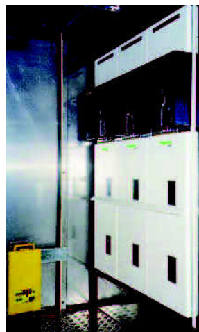
Installation of 400 - 630 A units on a 350 mm plinth
