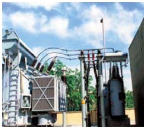
20kV outdoor termination used in Iran
