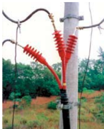
15kV outdoor termination used in Guangzhou
