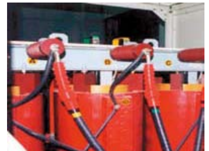
20kV indoor termination used in Iran
